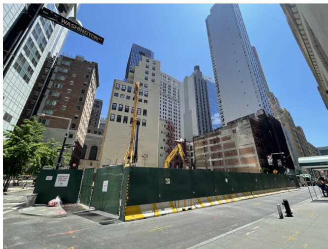
111 Washington Street development site (formerly 8 Carlisle Street)
