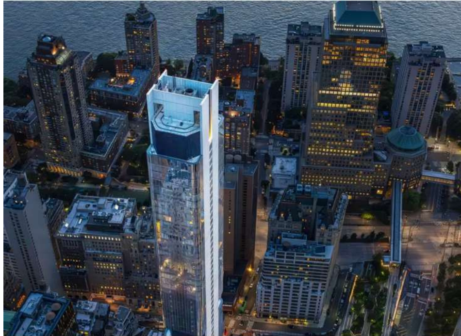
With 272 condo units, The Greenwich by Rafael Vinoly is one of the city's largest (and tallest) new development offerings
